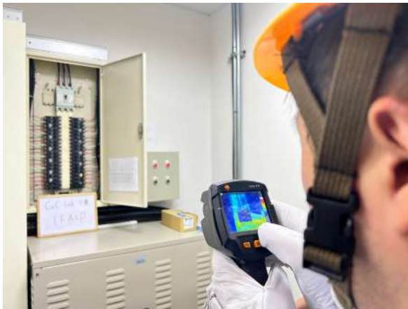
Infrared Electrical Panel Inspection
